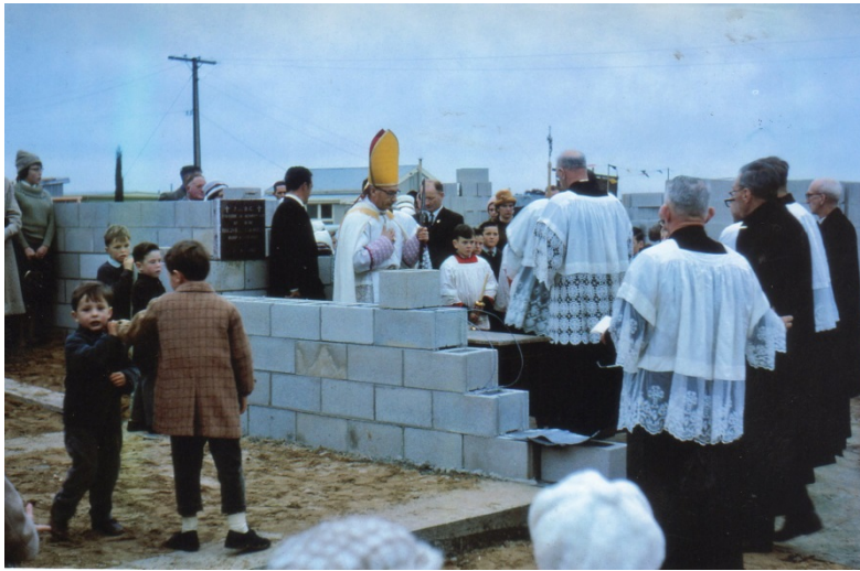
Bishop Bryan Gallagher assisted by priests from the Dioceses of Port Pirie and Adelaide, lays the foundation stone on July 14 th , 1963 and blessed the grounds where the new Church would be built.
